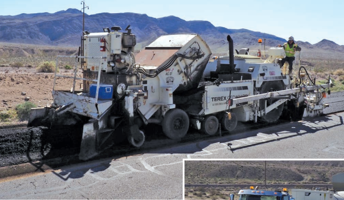
Left: Hat Creek Construction following the CIR Train on State Route 127 project utilizing their Bomag MS2 pickup machine and their Terex-Cedarapids 552 Asphalt Paver.
