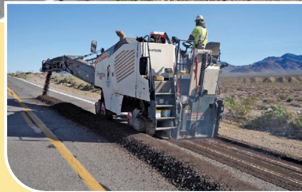
Right: PRS using a Wirtgen supplemental milling machine to pre-grind outside edge of asphalt pavement to increase paving width to 16 feet.
