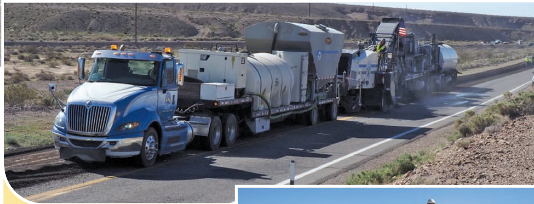
Right: PRS using a Wirtgen supplemental milling machine to pre-grind outside edge of asphalt pavement to increase paving width to 16 feet.
